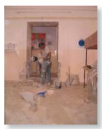
We made use of the summer holidays to do some necessary renovations which included a first aid room, and two additional wash rooms, besides the maintenance of the old ones. The wooden partition between class one and two was replaced by a concrete wall for sound proof purposes, and new windows were installed in that section.
